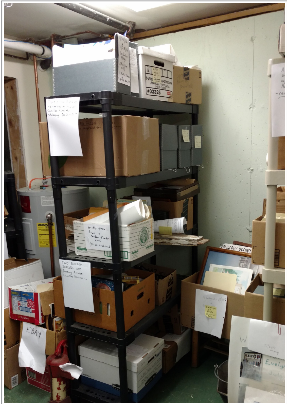
Pipes and sprinklers directly over shelves pose a risk of water damage to the items stored below.
