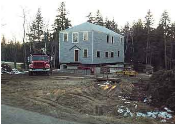
Cranberry House being moved onto foundation
