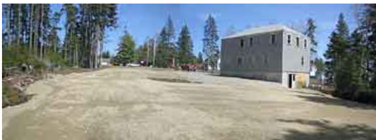
Cranberry House (rear view) and driveway to Main Road (photo taken from back of parking lot)
